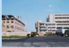
TBR Plant in Xiasha
